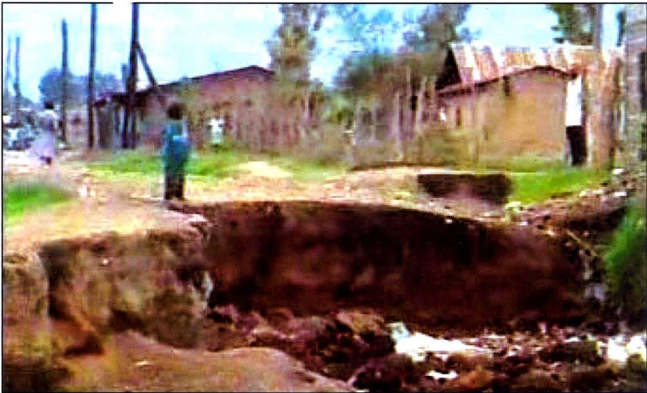
Picture1: photograph showing land subsidence
