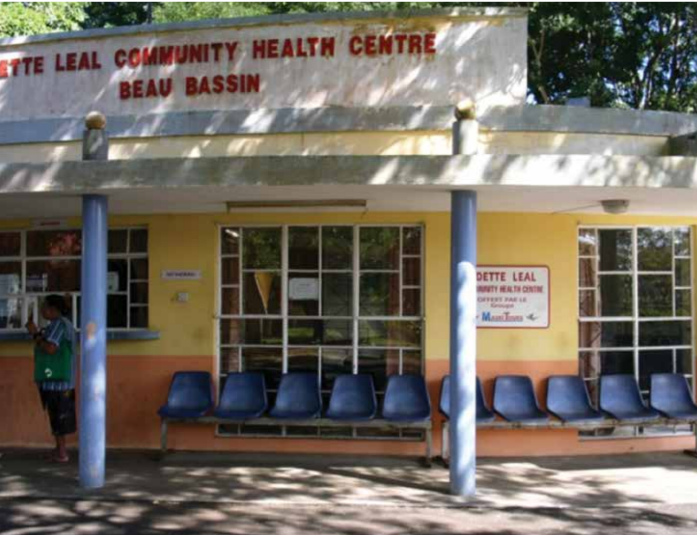
Community health centre in Mauritius. WHO
