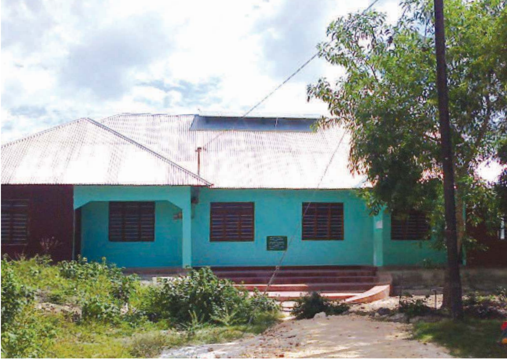
Solar panel installed to support Kijini PHCU services
