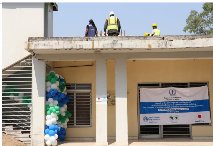
Launching of the the second phase construction of the Public Health Emergency Operation Centre
