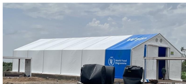
Figure 6: New isolation site Rub-Hall tent donated by WFP to support EVD readiness in Juba
