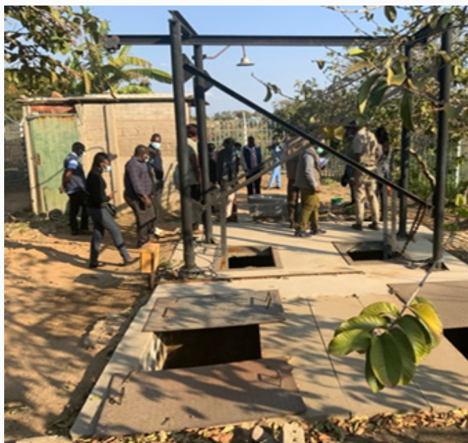
PHEOC, WHO and Bulawayo City assessing a point where sewer pumping is done which was reported to be malfunctional
